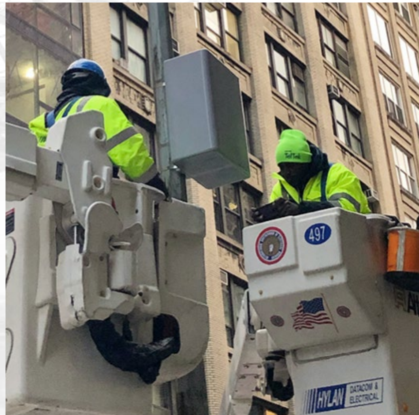
Mobile telecommunications workers in New York install a shroud for 5G equipment
